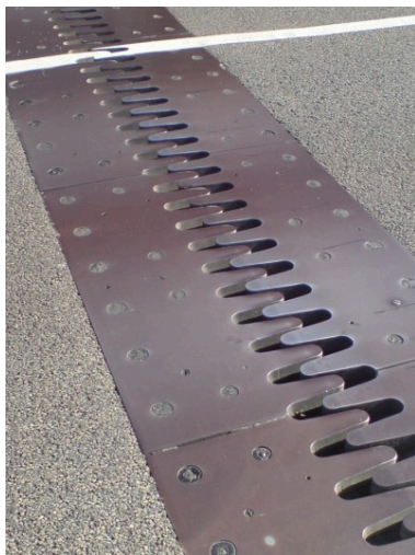
Figure 1. Thermal expansion joints like these in the Auckland Harbour Bridge in New Zealand allow bridges to change length without buckling. (credit: Ingolfson, Wikimedia Commons)
