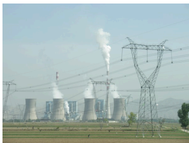
Figure 3. Tremendous amounts of electric power are generated by coal-fired power plants such as this one in China, but an even larger amount of power goes into heat transfer to the surroundings. The large cooling towers here are needed to transfer heat as rapidly as it is produced. The transfer of heat is not unique to coal plants but is an unavoidable consequence of generating electric power from any fuel—nuclear, coal, oil, natural gas, or the like. (credit: Kleinolive, Wikimedia Commons)
