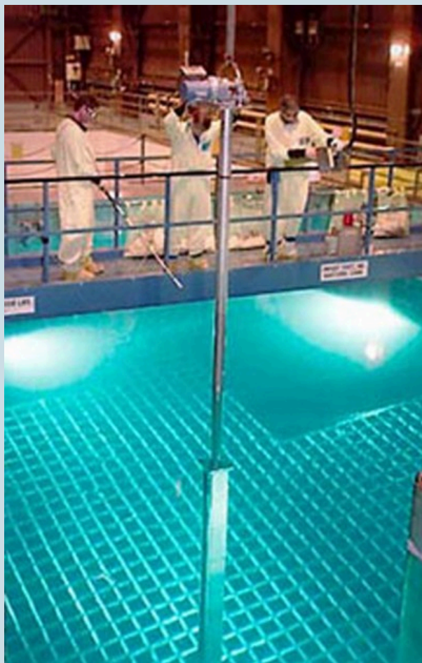
Figure 3. Radioactive spent-fuel pool at a nuclear power plant. Spent fuel stays hot for a long time. (credit: U.S. Department of Energy)
