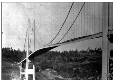
Figure 4. In 1940, the Tacoma Narrows Bridge in Washington state collapsed. Heavy cross winds drove the bridge into oscillations at its resonant frequency. Damping decreased when support cables broke loose and started to slip over the towers, allowing increasingly greater amplitudes until the structure failed (credit: PRI's Studio 360, via Flickr)
