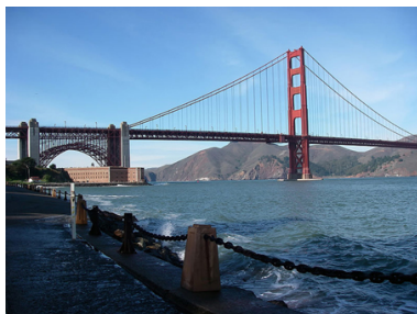
Figure 9. Unless an infinite tension is exerted, any flexible connector—such as the chain at the bottom of the picture—will sag under its own weight, giving a characteristic curve when the weight is evenly distributed along the length. Suspension bridges—such as the Golden Gate Bridge shown in this image—are essentially very heavy flexible connectors. The weight of the bridge is evenly distributed along the length of flexible connectors, usually cables, which take on the characteristic shape. (credit: Leaflet, Wikimedia Commons)
