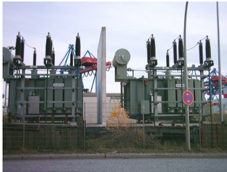
Figure 4. Power is distributed over large distances at high voltage to reduce power loss in the transmission lines. The voltages generated at the power plant are stepped up by passive devices called transformers (see Transformers ) to 330,000 volts (or more in some places worldwide). At the point of use, the transformers reduce the voltage transmitted for safe residential and commercial use. (Credit: GeorgHH, Wikimedia Commons)
