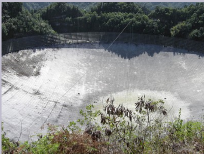
Figure 4. A 305-m-diameter natural bowl at Arecibo in Puerto Rico is lined with reflective material, making it into a radio telescope. It is the largest curved focusing dish in the world. Although D for Arecibo is much larger than for the Hubble Telescope, it detects much longer wavelength radiation and its diffraction limit is significantly poorer than Hubble's. Arecibo is still very useful, because important information is carried by radio waves that is not carried by visible light. (credit: Tatyana Temirbulatova, Flickr)
