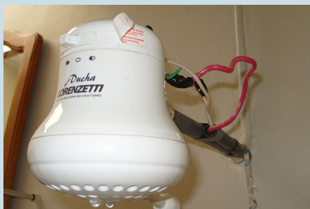
Figure 3. On-demand electric hot water heater. Heat is supplied to water only when needed. (credit: aviddavid, Flickr)
