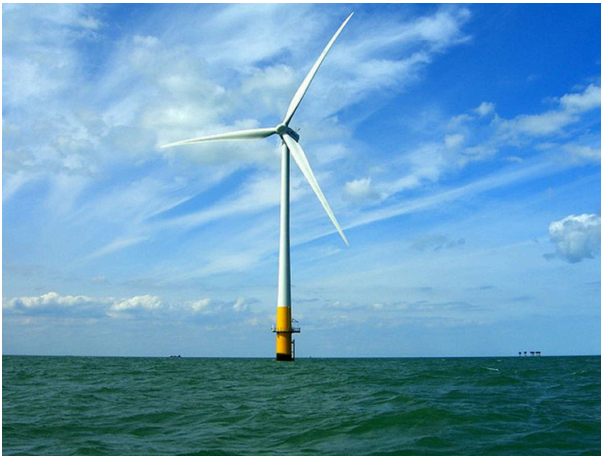
Figure 1. This wind turbine in the Thames Estuary in the UK is an example of induction at work. Wind pushes the blades of the turbine, spinning a shaft attached to magnets. The magnets spin around a conductive coil, inducing an electric current in the coil, and eventually feeding the electrical grid. (credit: phault, Flickr)
