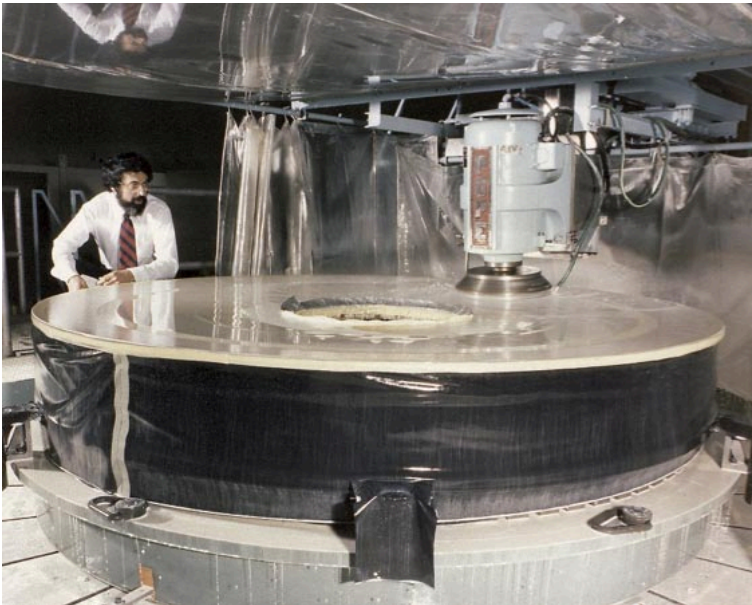
Grinding of the Hubble Space Telescope Mirror, 1979Public Domain |
