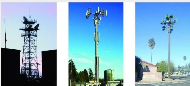
Figure 3. Radio and cell towers are typically used to transmit long-wavelength electromagnetic radiation. Increasingly, cell towers are designed to blend in with the landscape, as with the Tucson, Arizona, cell tower (right) disguised as a palm tree. (credit left: modification of work by Sir Mildred Pierce; credit middle: modification of work by M.O. Stevens)
