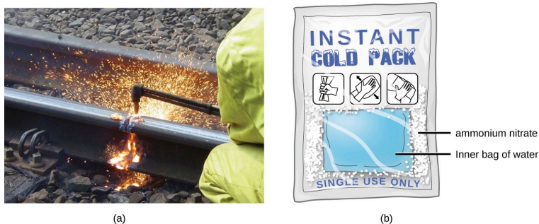
Figure 6. (a) An oxyacetylene torch produces heat by the combustion of acetylene in oxygen. The energy released by this exothermic reaction heats and then melts the metal being cut. The sparks are tiny bits of the molten metal flying away. (b) A cold pack uses an endothermic process to create the sensation of cold. (credit a: modification of work by “Skatebiker”/Wikimedia commons)
